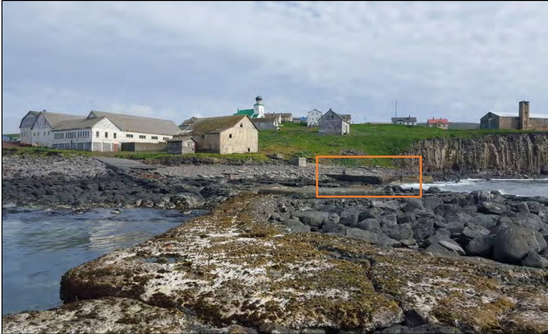
Figure 8. View of St. George Village from XPI-194. The inside landing (XPI-195) is on the right in the orange outline. The Seal Skin Plant (XPI-018) is the large white building on the left, while the Great Martyr Orthodox Church (XPI-004) is uphill near the center (Sparaga 2018).
