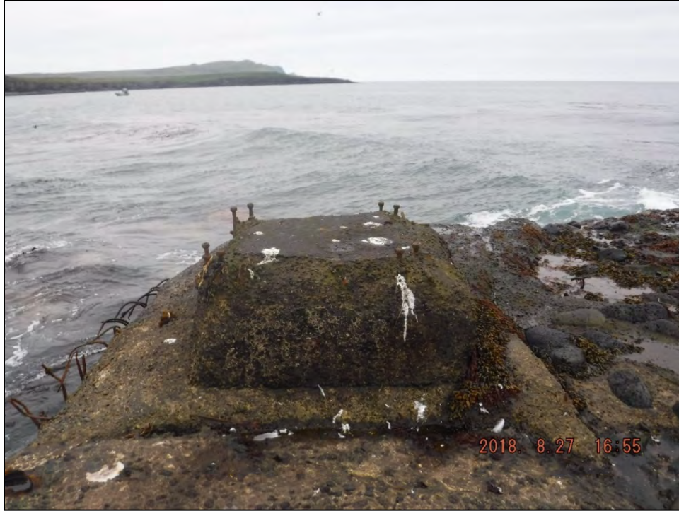
Figure 15. Concrete and metal object at the end of the St. George Outside Landing (XPI-194); this would likely have supported a boom lever attached to unload supplies from boats (Sparaga 2018).
