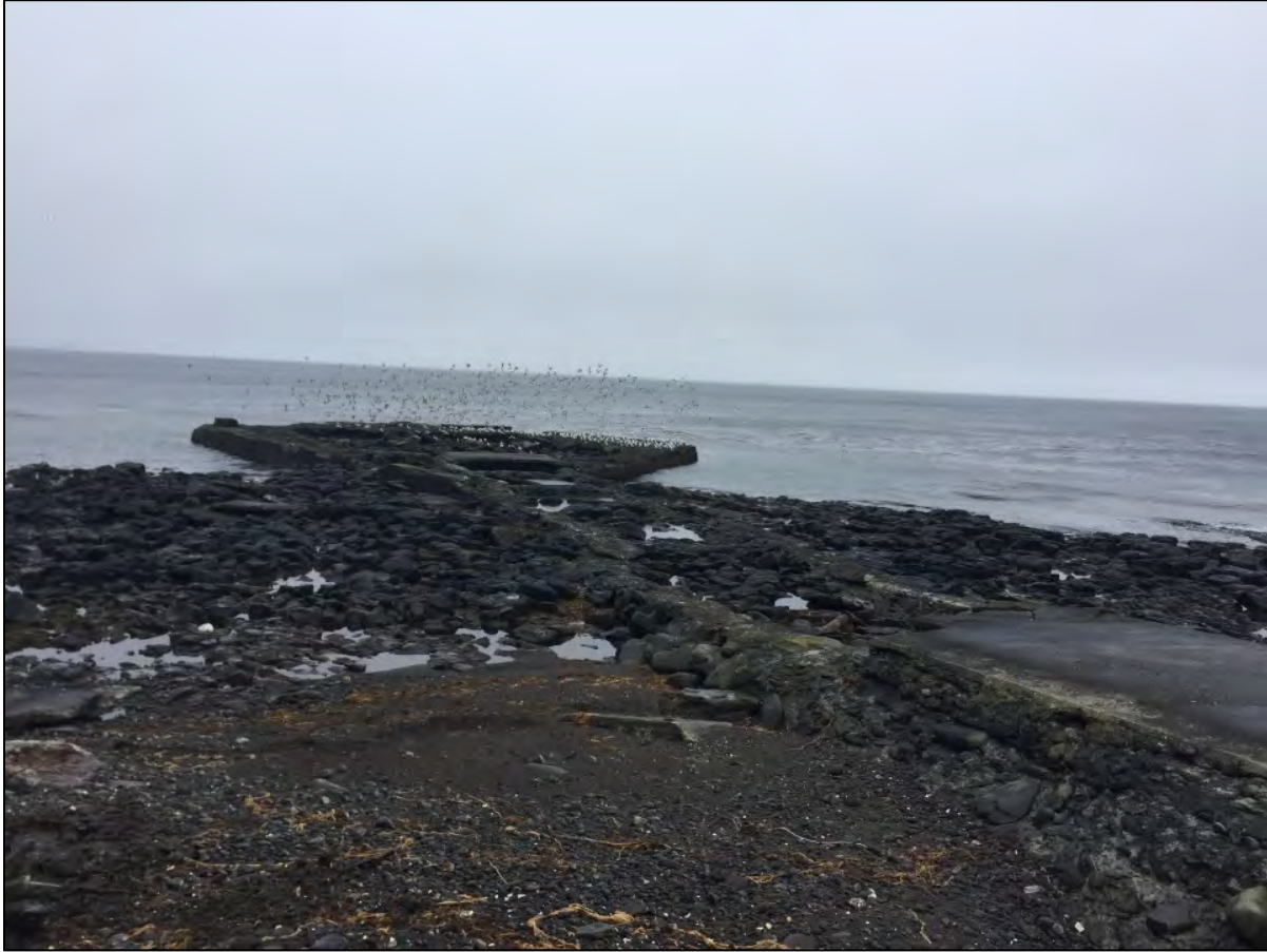
Figure 5. St. George's derelict small boat landing area.
